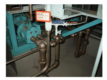
Showing sample valve on return line. While off the side of a vertical portion of the main line and after an elbow it is actually on a deadheaded line to a pressure gauge and is taken off of the bottom of the sample line. Not good.
