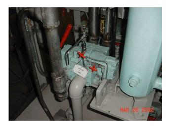
Showing sample valve on the return line. Valve is at the inlet to the directional valve in the top of the housing shortly after an elbow. Better location.
