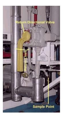
Showing sample valve on return line. Location is on a long dead headed line to a pressure gauge and after a long vertical down leg of the main line. Not good.
