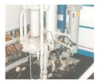
Showing sample valve on return line. Valve is at the top of an elbow on the supply to the directional valve and it has a long goose neck. This goose neck should not be inserted into the sample bottle.
