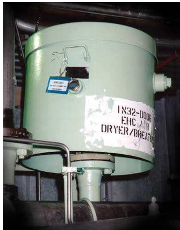
Figure 2. Standard Desiccant Breather Used on a GE Reservoir
